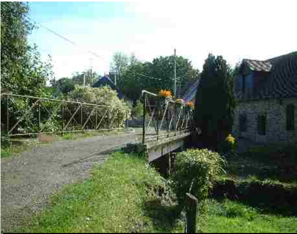
The bridge at le Plessis
